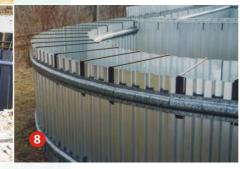
The 3.1 meter lightweight foundation wall shutter ing element adheres to its shape thanks to 27 vertical trapezoidal profiles.
