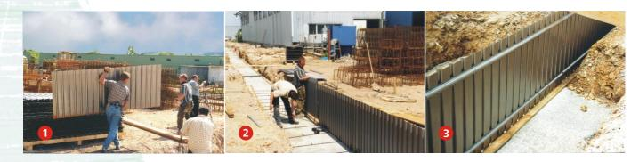
MSL FS 2001 foundation shuttering consists of only two components. 1) Foundation wall shuttering element 2) Insertible connector
